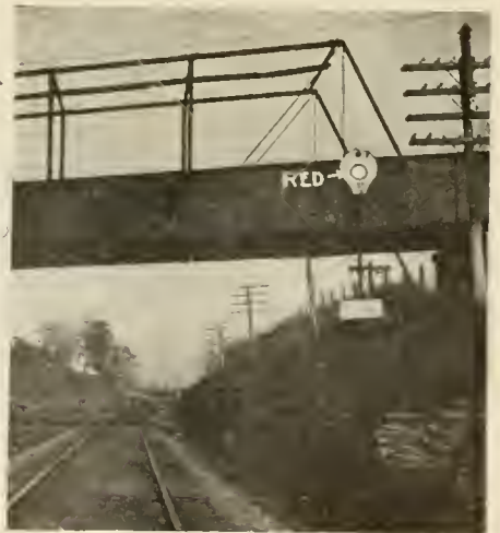
FIG. 7. BLOCK SIGNAL DISC. COLOR TAKES PLACE OF POSITION
